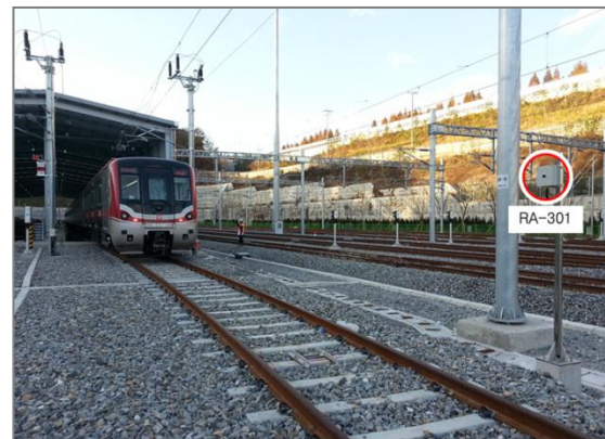
[RA-301 installed on a train pole]
